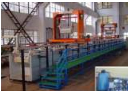
Electro Galvanizing Unit (UNIT 3)
